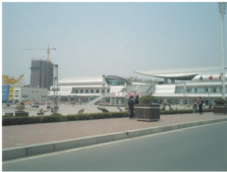
Development zone train station
