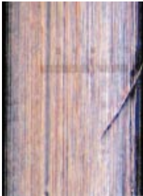
図9 特異き裂 Surface crack
